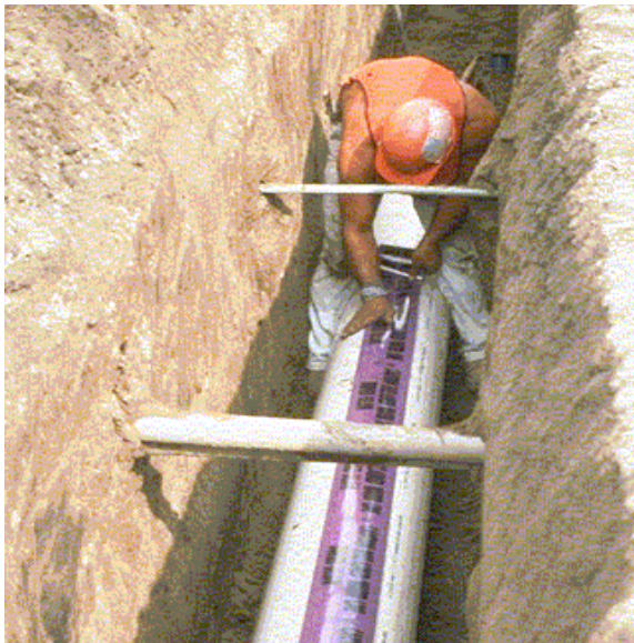
Recycled water pipeline installation with continuous purple warning tape
